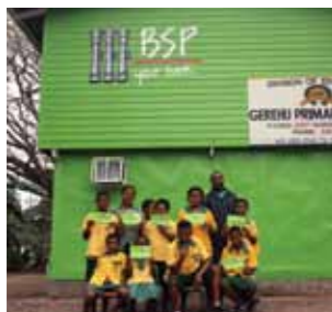
Gerehu Primary School Library Refurbishment - wire, air conditioner, book shelves, desks & painted building.
