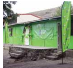
Kilakila Elementary School classroom & Admin O'ce Renovation - painted building, presented school materials.
