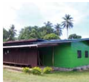
Dapu Health Clinic - constructed new extension for client waiting area with seating benches.
