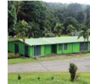
Kerevat CIS Admin Office Renovation - new flywire & curtains, internal repairs, full building repaint.
