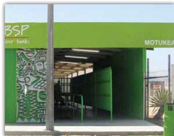
BSP Motukea - Containerized branch.
