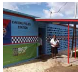
Kavieng Police Station - new internal fittings, louvres, floor tiles, fans, enquiry counter & new furniture.
