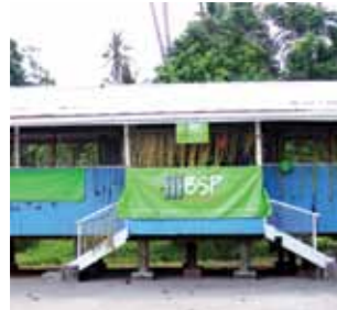
Nuwok Elementary School - repainted a double classroom and installed a new 5000L tu'a tank.
