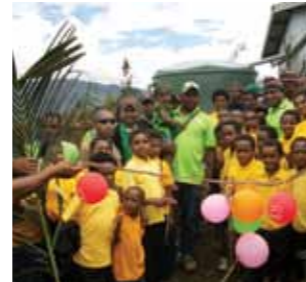
Kutubu Secondary School / Lumbi Primary School - installed 2 x new 5000L and 1x 9000L tu'a tanks.
