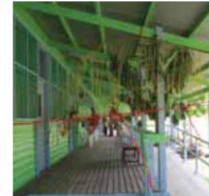
Kiunga Hospital Renovation - new flywire & curtains, internal repairs, full building repaint.
