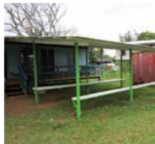
Daru Urban Clinic - reconstructed & extended new overhead shelter for patients.
