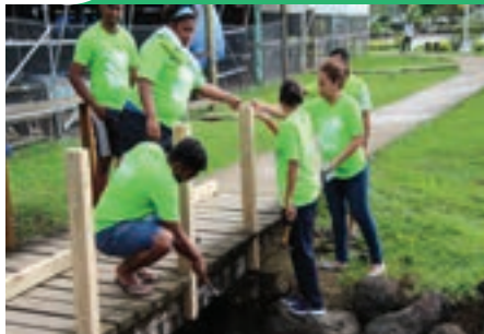
SAVUSAVU BRANCH Maintenance and refurbishment of bridge walkway.
