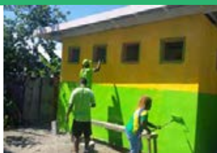
RANADI Lunga School Ablution Block renovation
