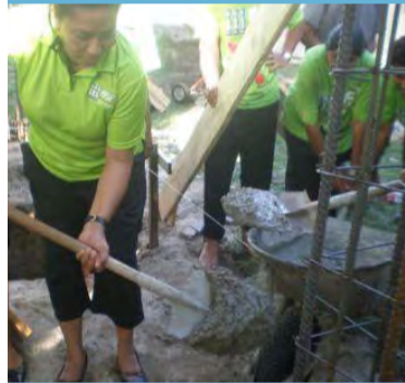
NEW WATER TANKS FOR CUVU COLLEGE
