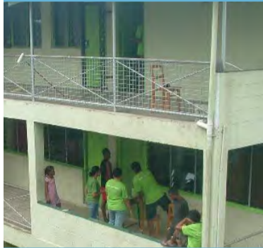
REPAINTING AND RENOVATION OF THE GOSPEL SCHOOL FOR THE DEAF
