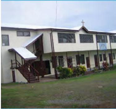
ST TERESA’S CATHOLIC SCHOOL REPAINTING AND RENOVATION
