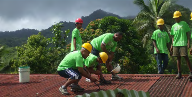
REPLACED OLD ROOFING IRON AT NAMOSI SECONDARY SCHOOL
