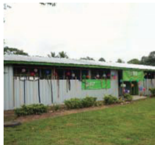
Hayfield Primary School - replaced external walls and painted Grade 5 double classroom building.
