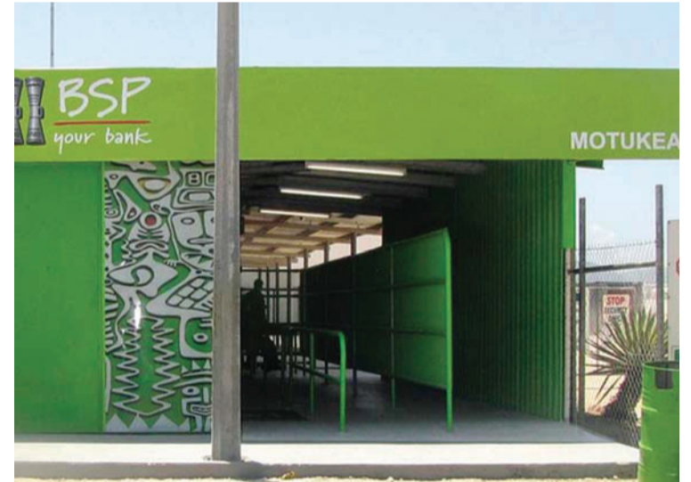
BSP Motukea - Containerised branch
