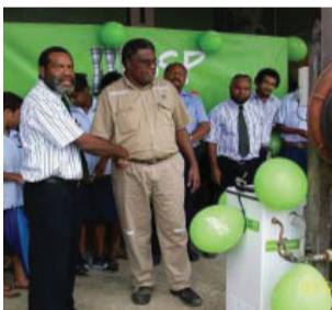
Tabubil High School - installed 3 new water coolers for the school after the old coolers posed health risks.
