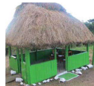
Tavua Muslim School - renovation classroom by BSP Tavua Branch
