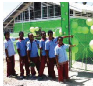
Koki Primary School Ablution Block Renovation - Replaced toilet doors, seats, pots & painted building.
