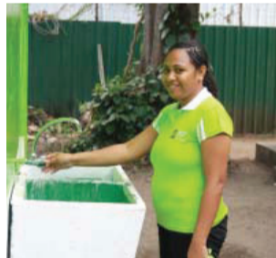
Konedobu Health Clinic - reconstructed ablation block, repaired flywires, walls, painted the whole building.
