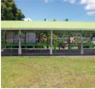
Omili Primary School - constructed the first new market building for parents to properly sell food to students.
