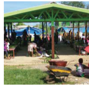
Bialla Town market - Constructed new market building for the locals to sell their product.
