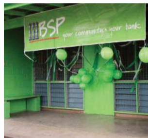
Bomana Police College Health Clinic - new flywire, curtains, internal repairs, full building repaint & presented new furniture.
