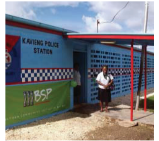
Kavieng Police Station - new internal fittings, louvres, floor tiles, fans, enquiry counter & new furniture.
