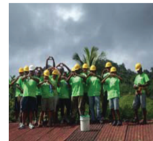
Namosi Primary School - renovation of school classroom by BSP Pacific House Branch
